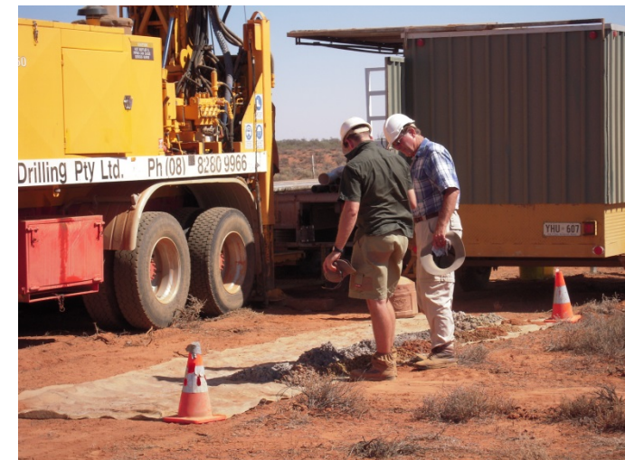
2009 drilling at Mulyungarie
