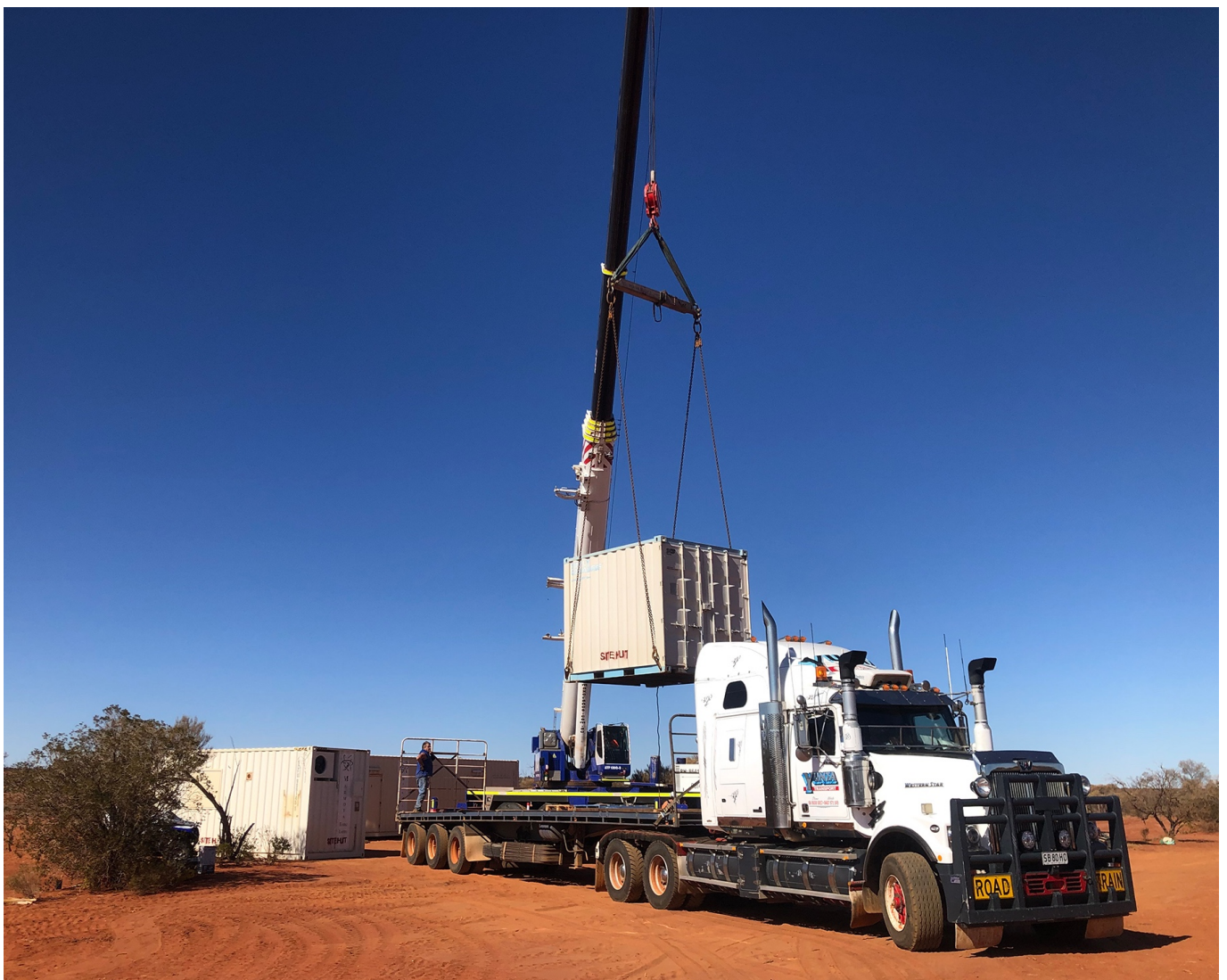
Figure 8: Components of camp being unloaded at Aurora Tank from road train
