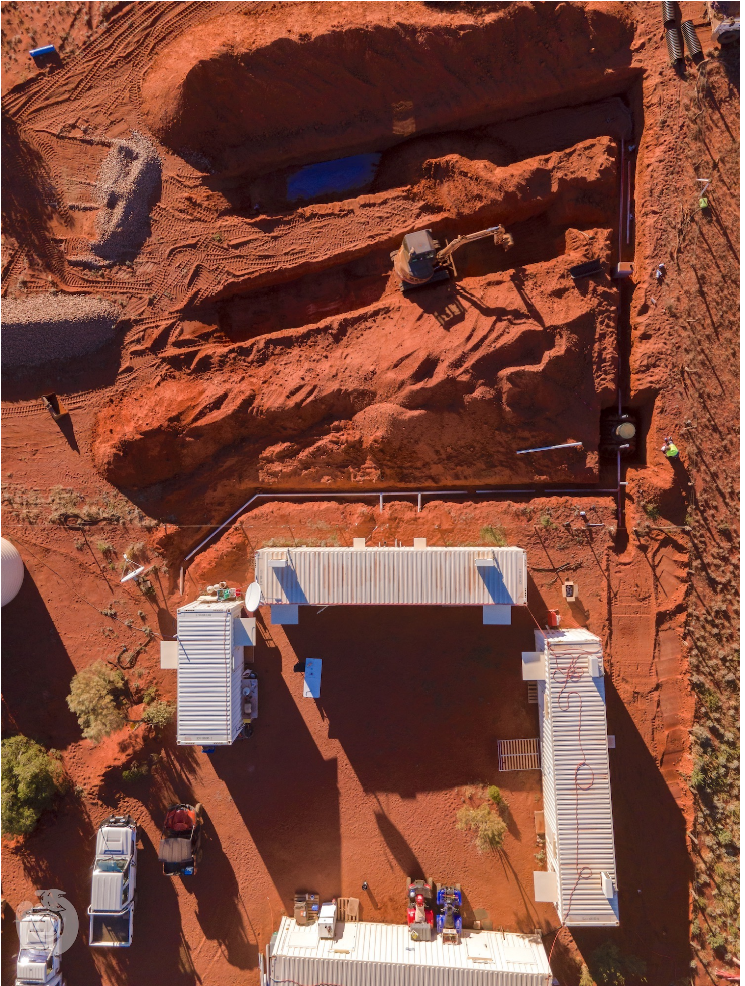
Figure 9: Aerial view of new infrastructure works (May 2021) at Aurora Tank camp
