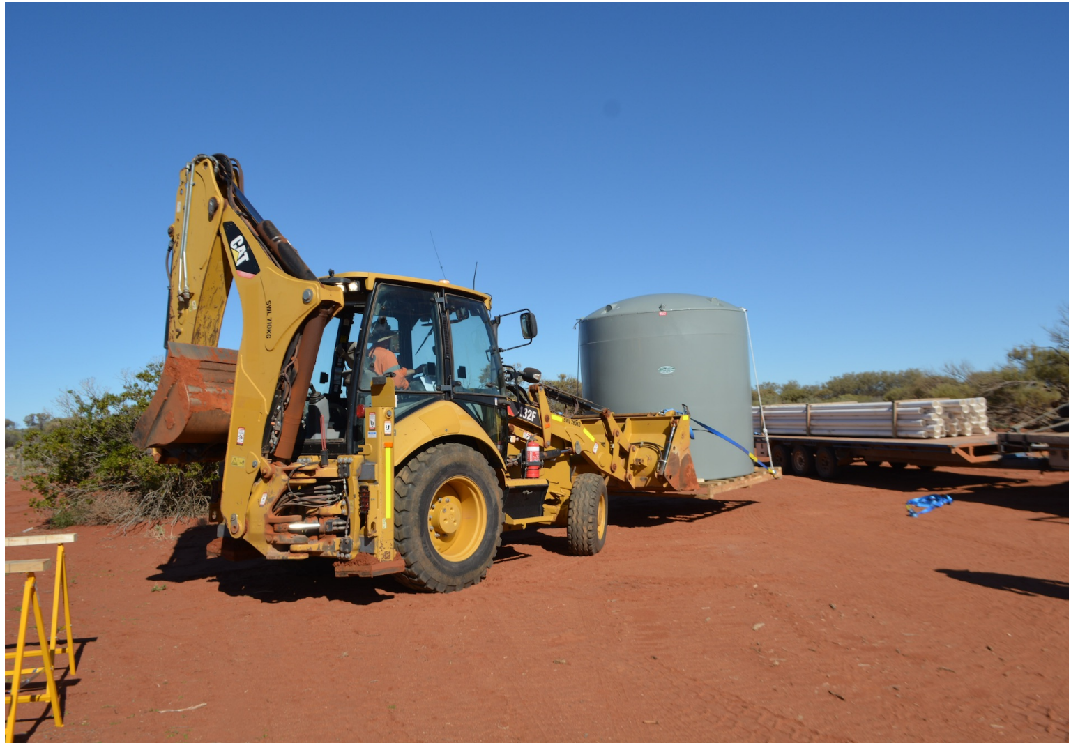
Figure 12: Self-bunded fuel tank arrives (June 2021)
